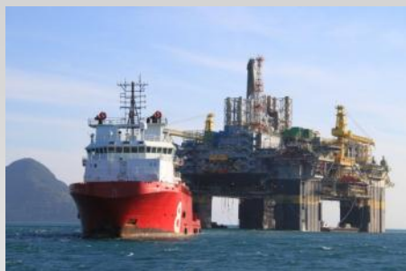
Production Platform P-56
